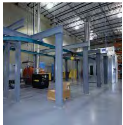
AREA 6: Paint Booth
